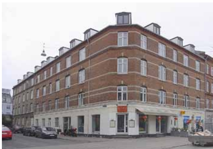
Facade mod gade
