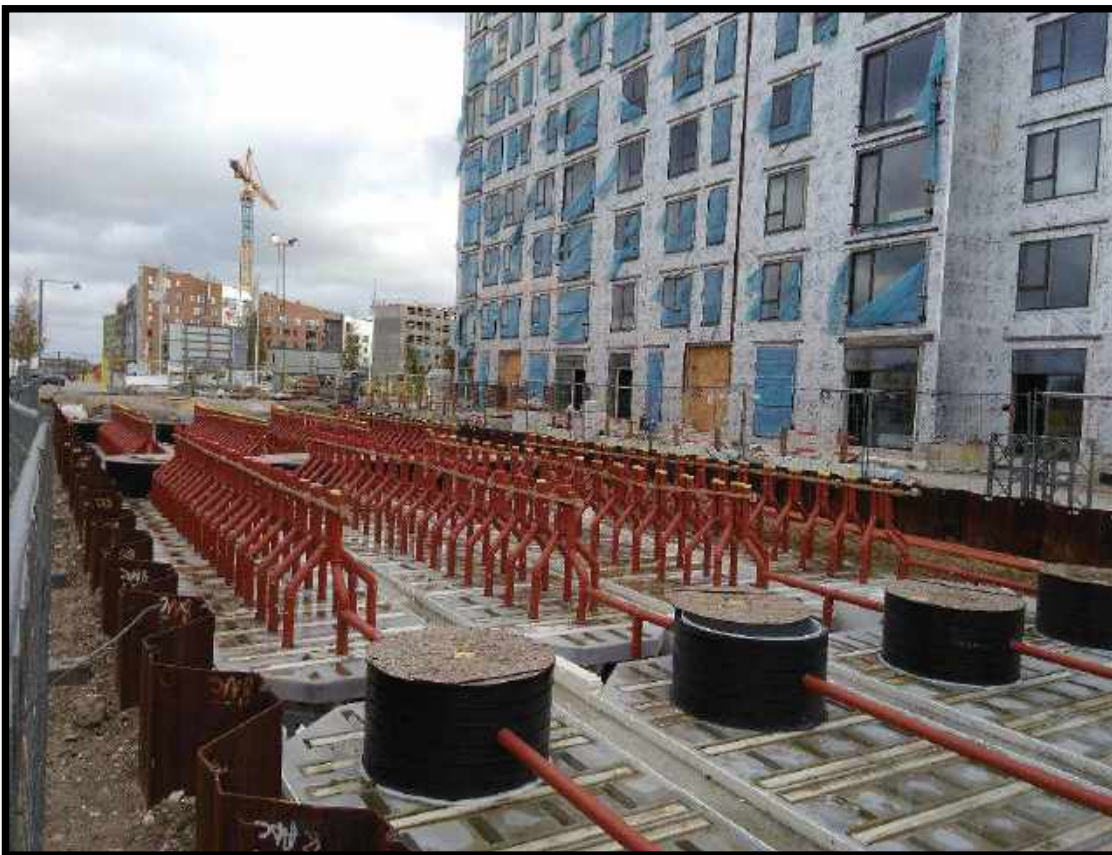
Figure 5: Dual Porosity Filtration Facility in Ørestad, prior to covering
