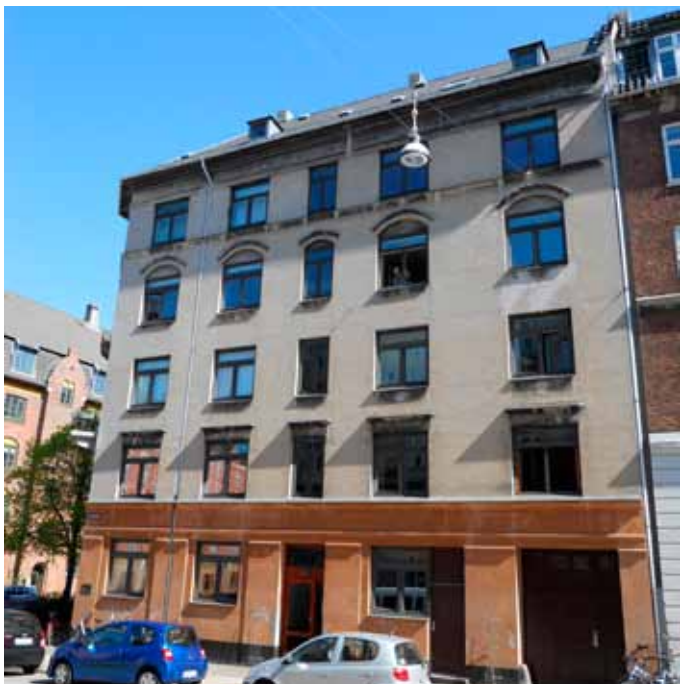
Facade mod Nannasgade
