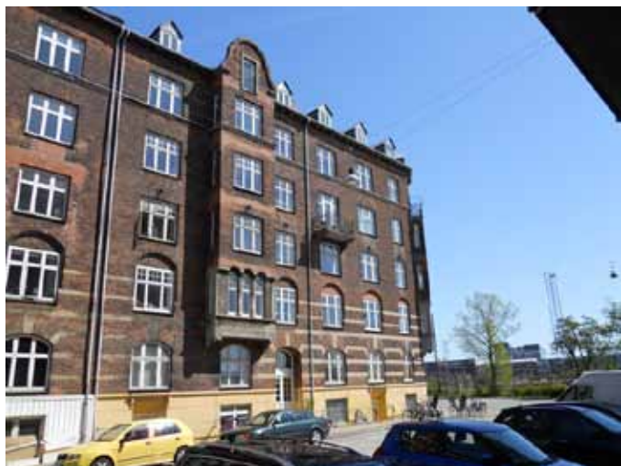
Facade mod Godsbanegade
