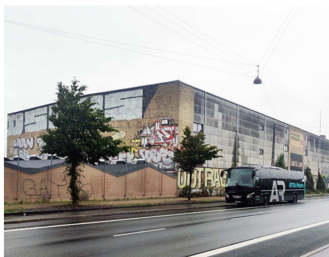
Rovsingsgade 68 set mod nord.
