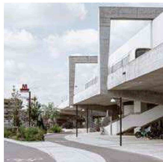
Det grønne loop under metroen, Orientkaj Station
