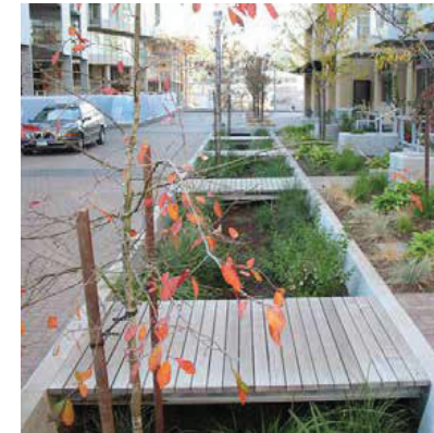
Regnvandsbed langs gade i Portland, USA
