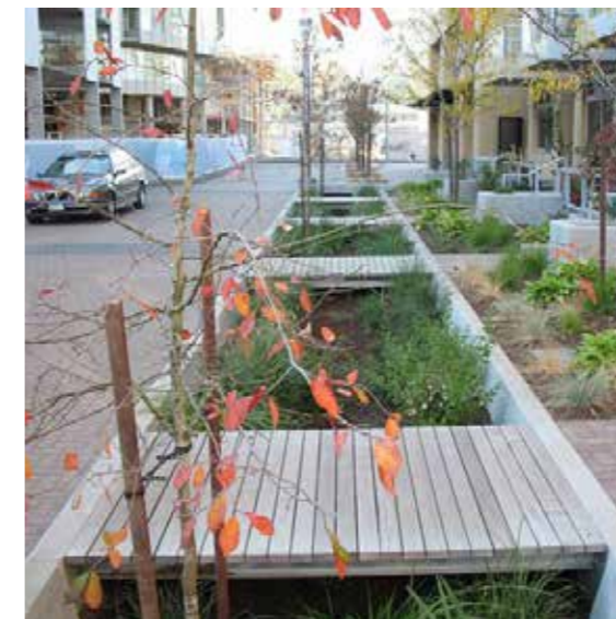
Regnvandsbed langs gade i Portland, USA
