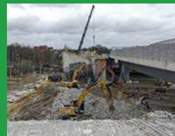
Deconstruction of the approximately 400-metre long Langenfelde Bridge
