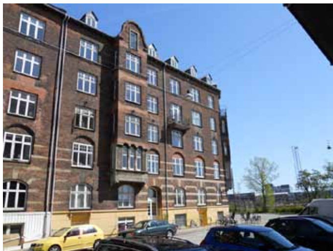
Facade mod Godsbanegade
