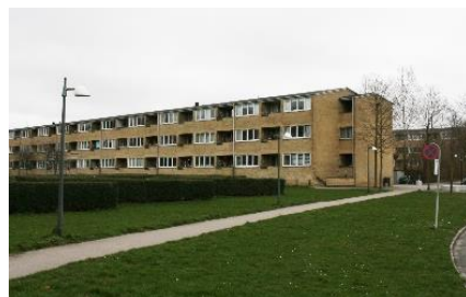
Facade mod have
