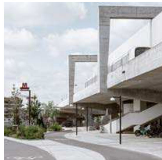
Det grønne loop under metroen, Orientkaj Station
