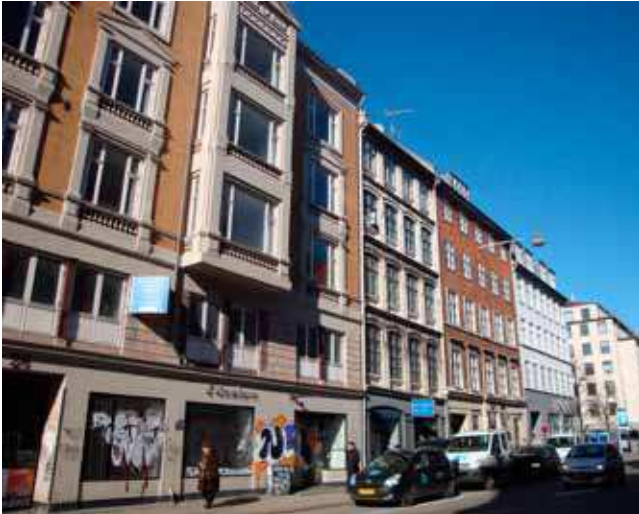
Facader mod Store Kongensgade.
