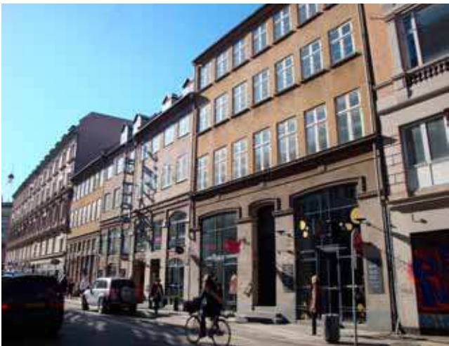
Facader mod Store Kongensgade.
