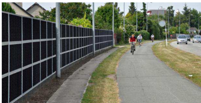
Figure 10: Miljøskærm's panels installed in residential area.
