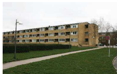
Facade mod have
