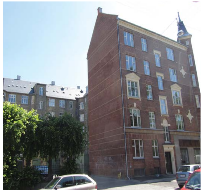
Facade mod Carlsgade
