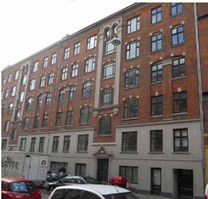
Facade mod Kronborggade
