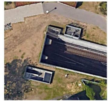
Figure 3: Portal Escape Stairs
