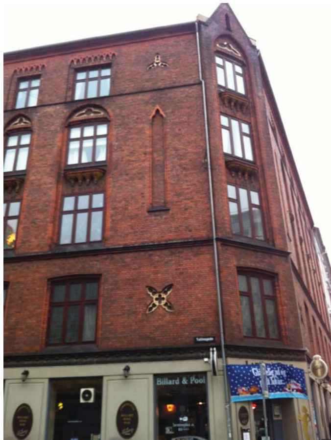
Facade mod Tullingsgade
