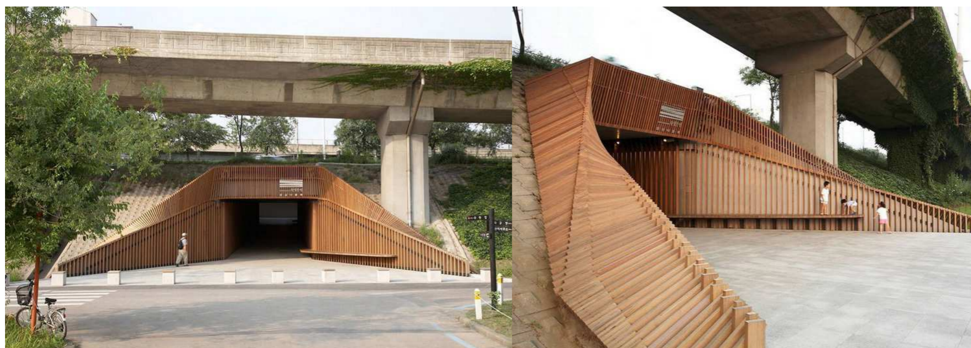
Seongsan Underpass, Seoul - LokalDesign
