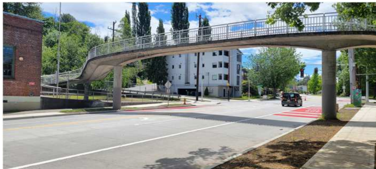
Delridge Pedestrian Bridge, Seattle
