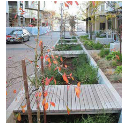
Regnvandsbed langs gade i Portland, USA
