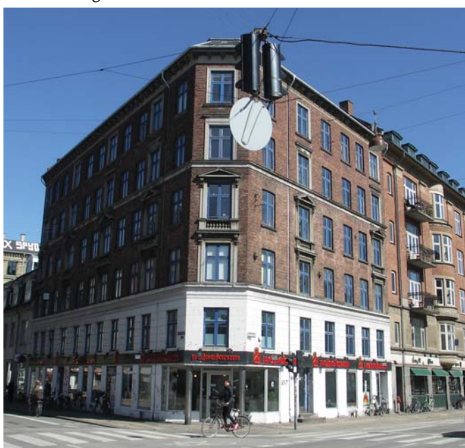
Facade mod gadeside
