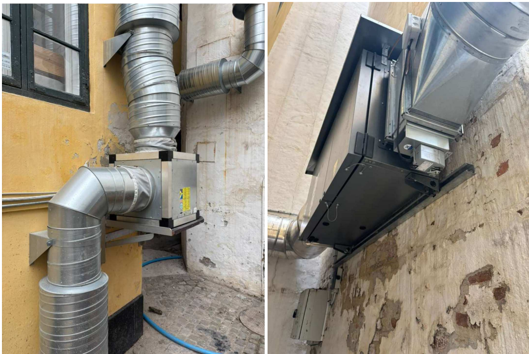
Figure 17: The cooling and ventilation system whose noise was measured at the Miljøpunkt Indre By & Christianshavn's office
