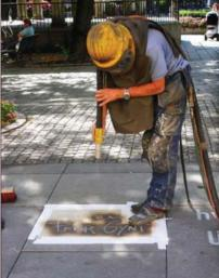
A quote of 30 letters can be done in a couple of hours. The compressor is not too loud and since the sand it's heavy, do not create a dust cloud.
