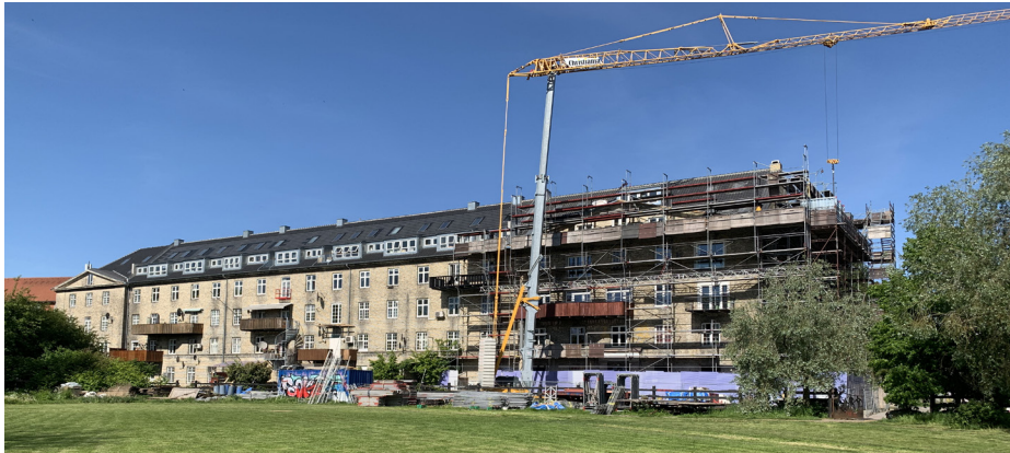
Fredens Ark under renovering
