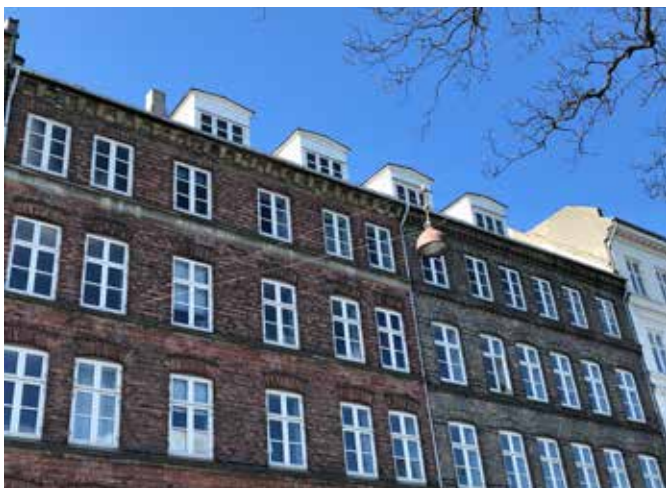
Facade mod gaden.
