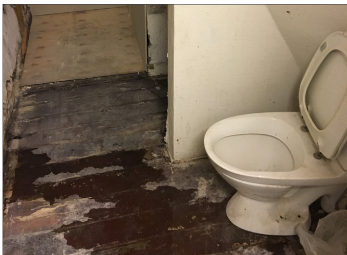
Wc under renovering.
