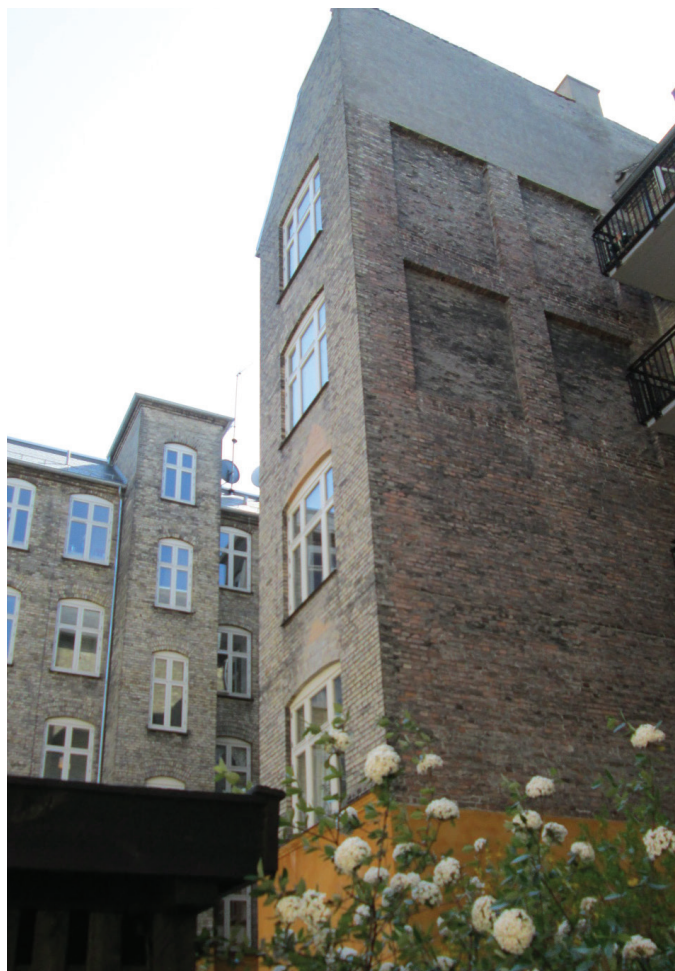
Facade mod gård
