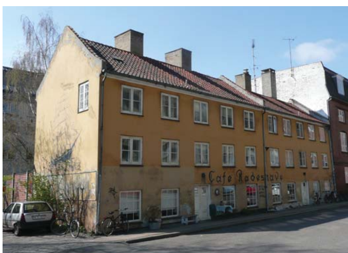
Facade mod Langebrogade
