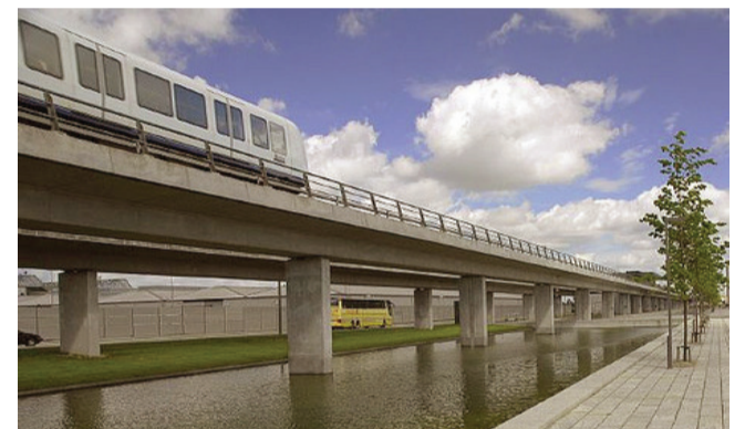
The close proximity to the Copenhagen metro is an important part of the project
