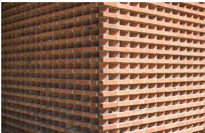
Referencefoto - Lindevang Transformestation. Illustration: GOTTLIEB PALUDAN ARCHITECTS
