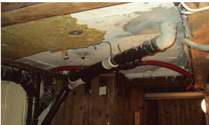
Manglende isolering
