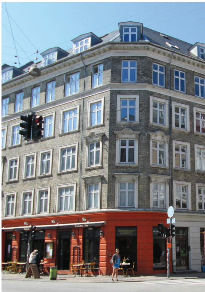
Facade mod gaden
