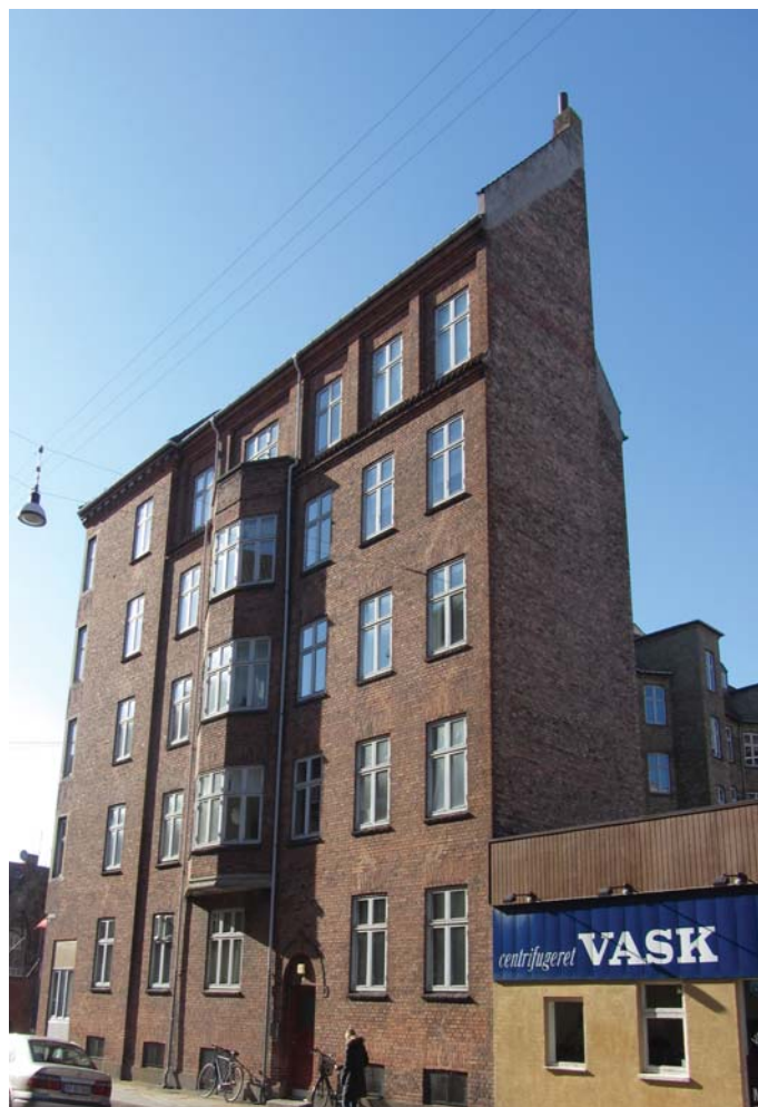
Facade mod Bulgariensgade. Gavl isoleres
