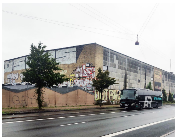
Rovsingsgade 68 set mod nord
