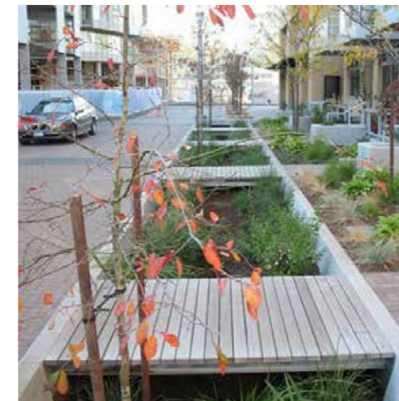
Regnvandsbed langs gade i Portland, USA
