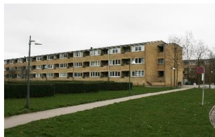
Facade mod have
